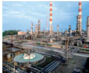
Oil and gas conveyance technology
